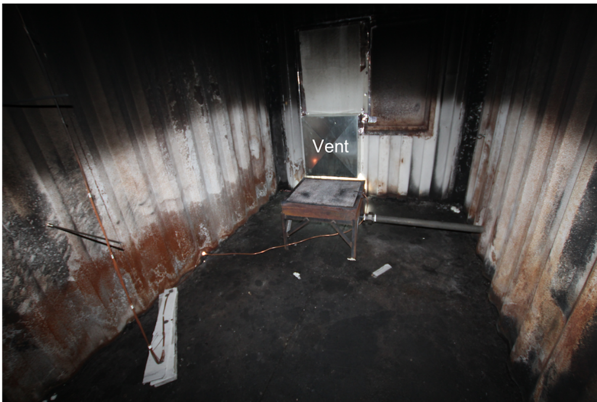
Figure 3.4: Photograph of propane burner installed in the fire room.
