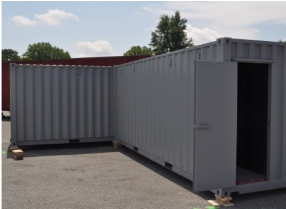
Figure 3.1: Exterior view of the test structure.
