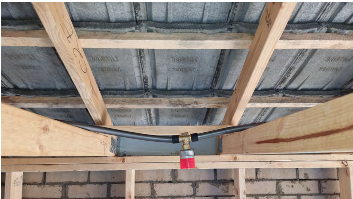
Figure 5-4. Sprinkler in roof space at rough-in (image from Shae Mete, 2024).
